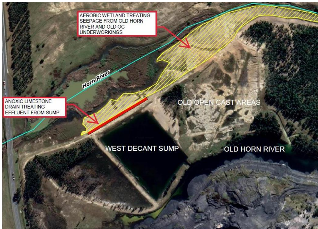
Figure 1-3: West Decant Sump area to be treated with ALD and cut off Aerobic Wetland along Horn River boundary
