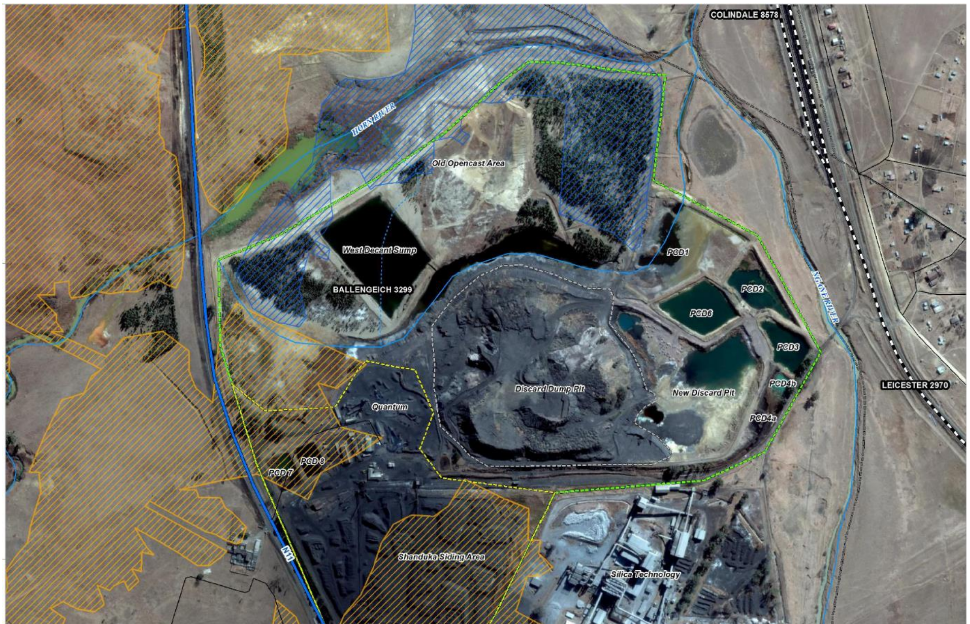
Figure 2: Ballengeich Mine Infrastructure Overview
